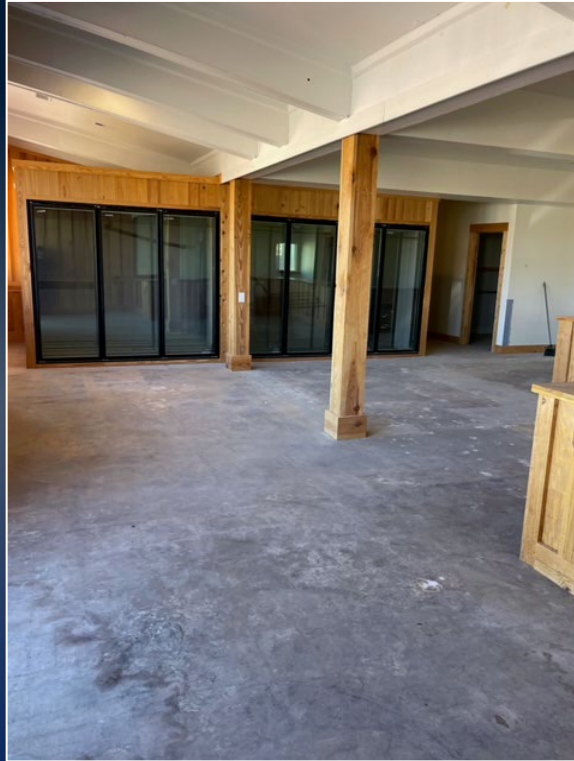
Building 1 – Walk-in Cooler
